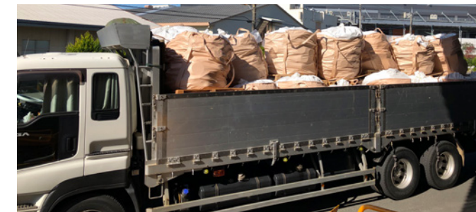
Recycled materials being carried out
