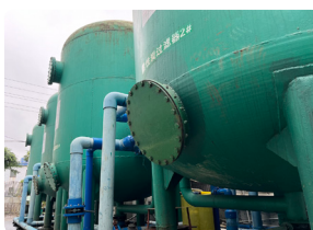
Final filtration tanks
