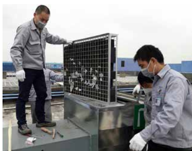
Carbon filter being installed to the outdoor exhaust equipment (China)
