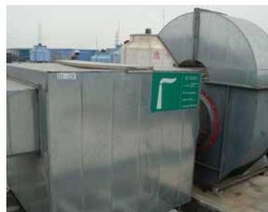
Carbon filter being installed to the outdoor exhaust equipment (China)
