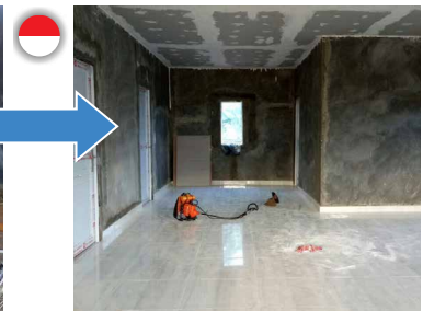
Construction was completed in October 2017
