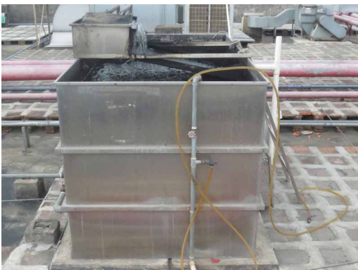
Filter for wastewater installed on the roof (China)
