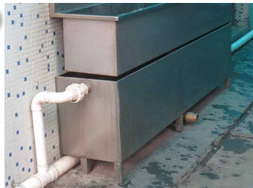
Device that collects wastewater from the lavatory and feeds it with a pump (China)
