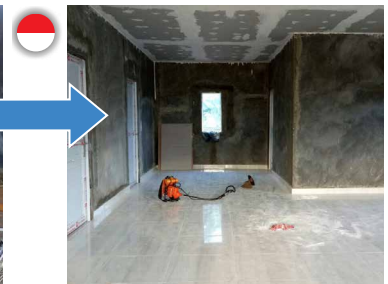
Construction was completed in October 2017
