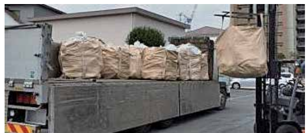
Recycled materials being carried out (headquarters)
