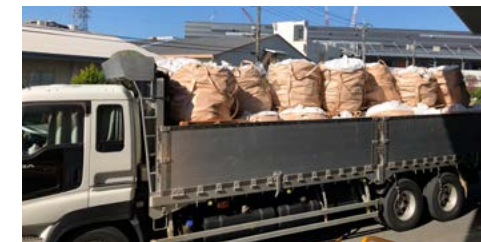
Recycled materials being carried out
