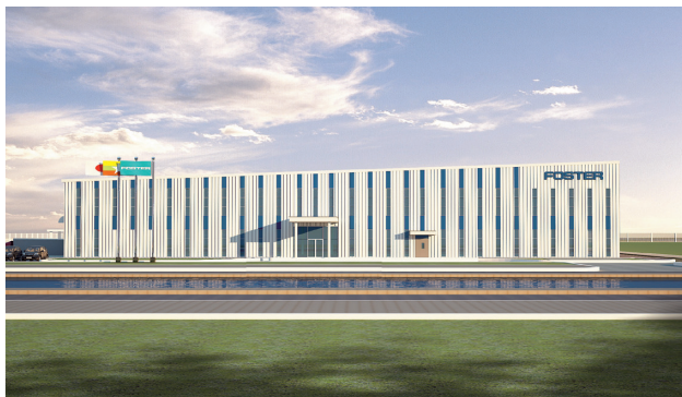
Image of the completed plant
